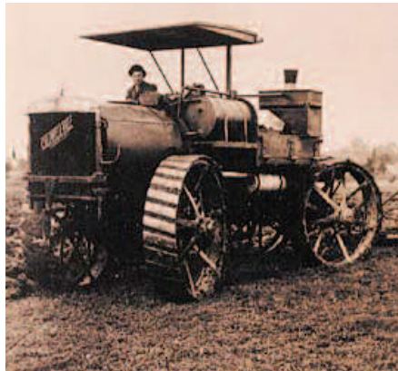
1910 80hp Caldwell Vale tractor featuring four wheel steering and an additional cooling tank on the rear to supplement the front radiator
